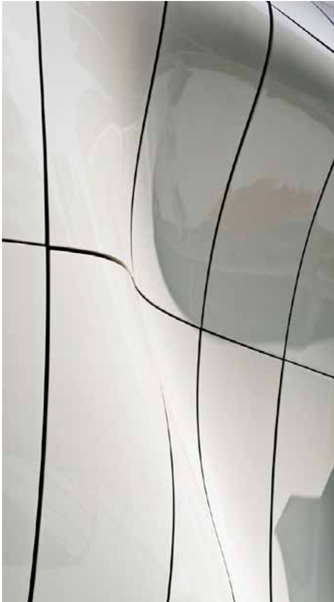
Figure 12.5: Detail of the FRP panels. Courtesy of Zaha Hadid Architects. Photograph: Virgile Simon.
